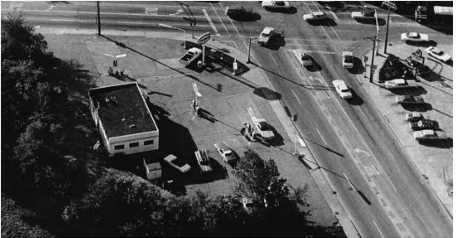
This is an aerial view of the intersection of Milwaukee Avenue and Dundee Road in Wheeling as seen in 1977.
