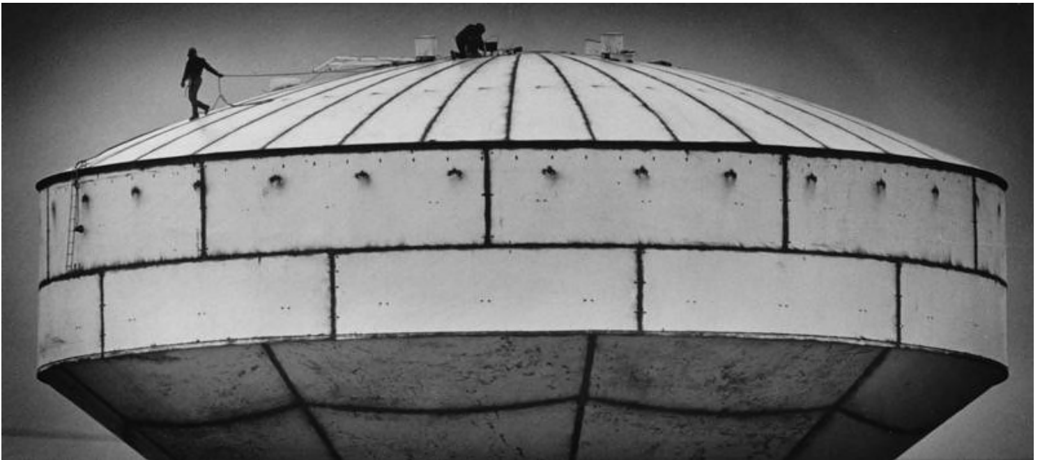
Construction workers weld the final pieces into place of the water tower on Wolf Road.
